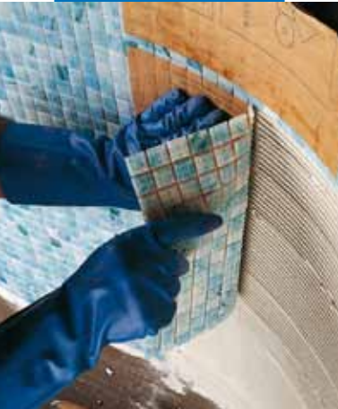
Glass mosaic 2x2 cm installation in a swimming pool with Adesilex P10 mixed with Isolastic diluted 1:1
